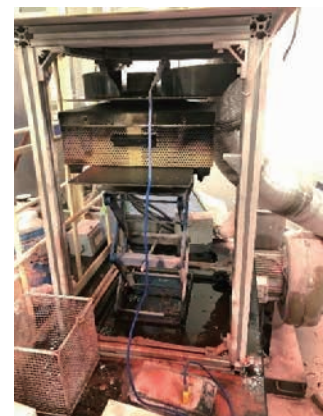
Around the oil-heating part
