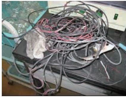
Burnt electrical wiring
