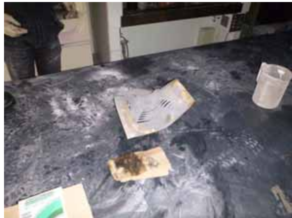
Plastic cover of ceiling speaker that was melted with heat
