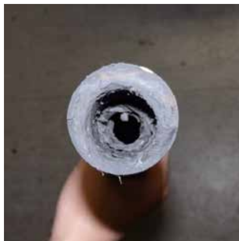
Inside of the vacuum hose
